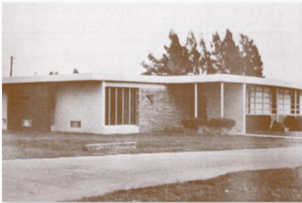
Completed Orlando Headquarters, 1970.
